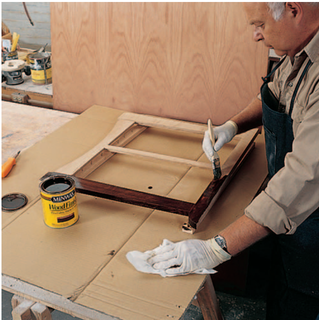
A well-applied coat of Minwax® dark walnut stain produces a reasonably close approximation to ammonia fuming. It's an appropriate tone for Arts & Crafts-styled pieces like this.
