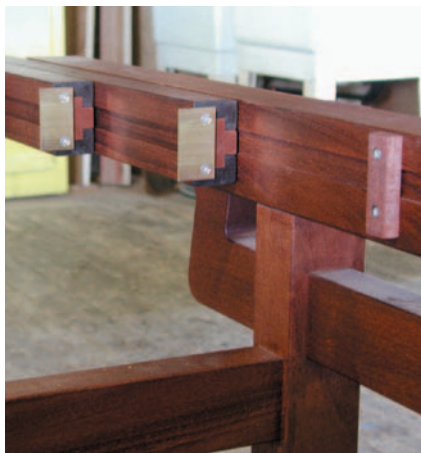
Brass closing plates are mounted as shown above. Also note the T-shaped stop blocks (pieces 12) secured with screws in the T-slots next to the closing block.
